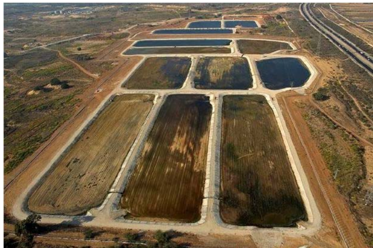
Figure 4 Infiltration basins at Yavne, Dan Region (Shafdan site)
