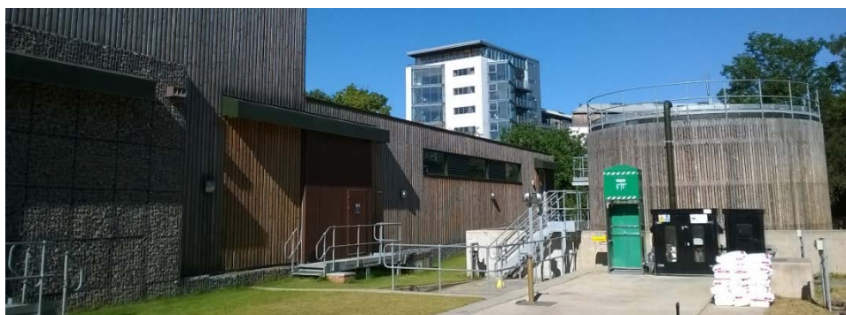
Figure 11 Old Ford water reclamation plant
