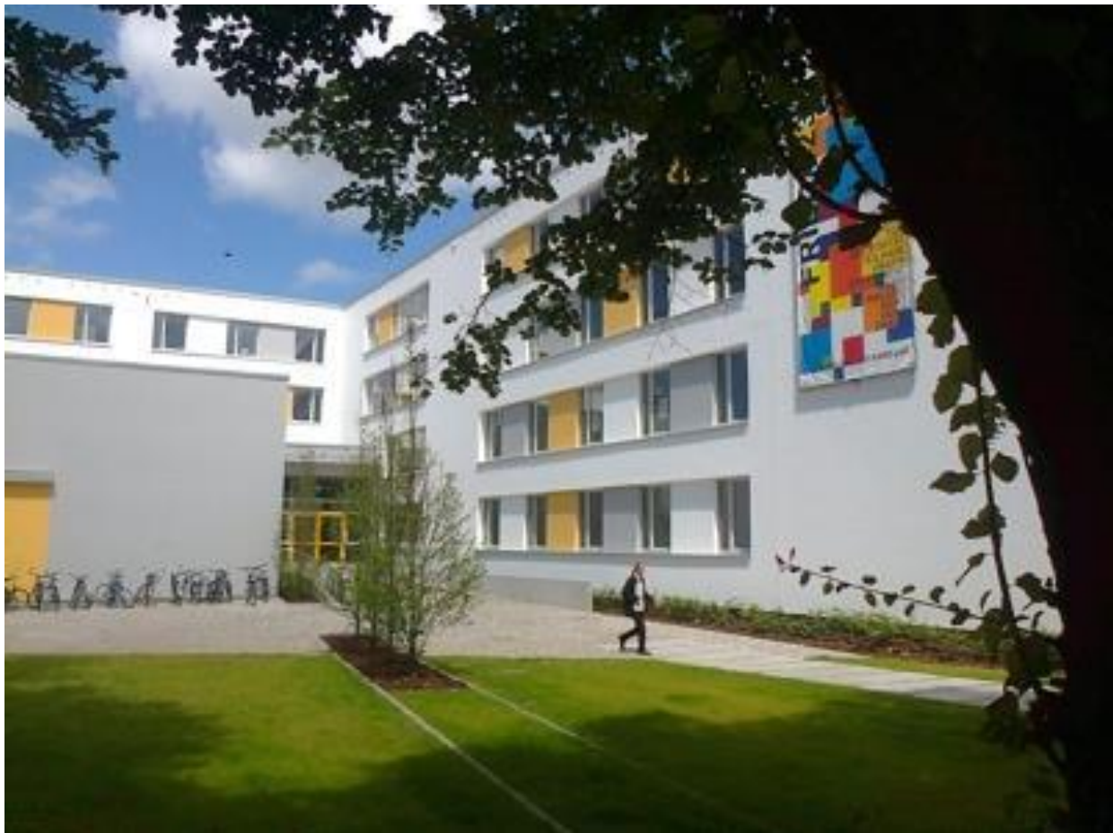
A transformed image of the Frieda 23 building
