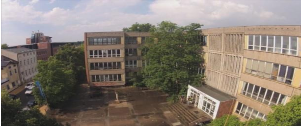
Image of the building before its transformation
