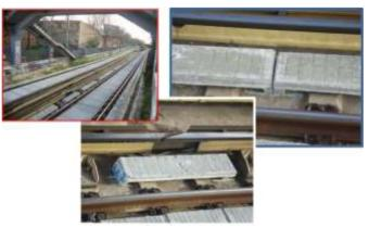
Figure 11: Absorbing track panels
