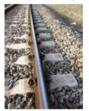
S<sub>3</sub> – HDS wide sleeper with wavy under sleeper pad
