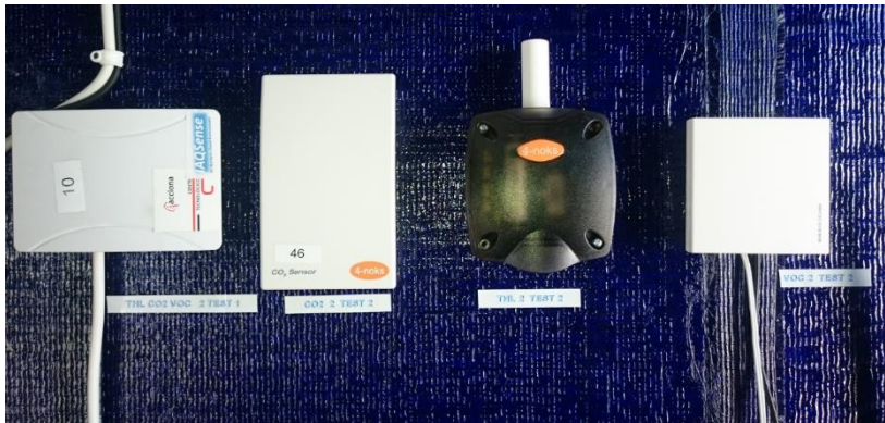
FIGURE 9 DETAILED PICTURE OF THE FIRST AND SECOND GENERATION SENSORS INSTALLED AT EACH LEVEL
