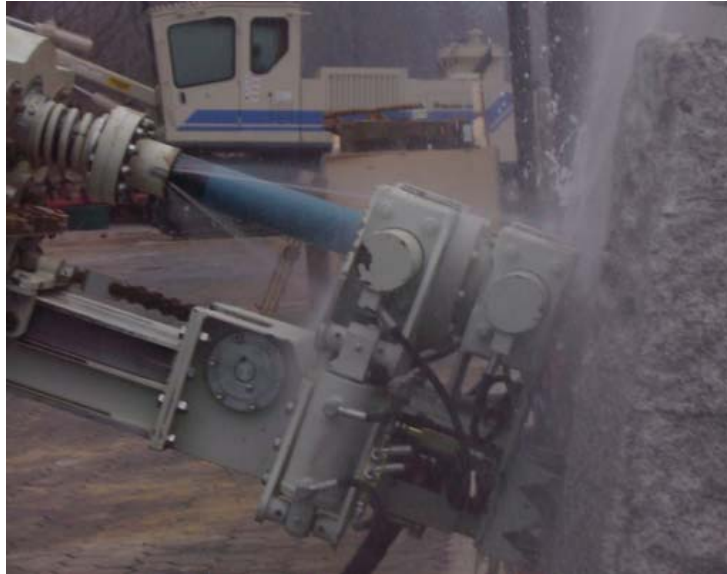
Figure 3-14: Water test on a pneumatic DTH hammer
