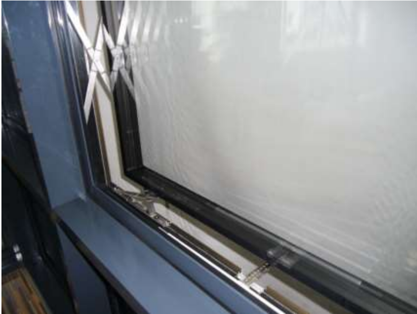
Figure 7: exemplary mounting of frameless, operable window in quadruple façade glazing
