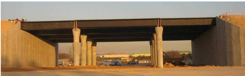
Figure 6. . Beams on their supports
