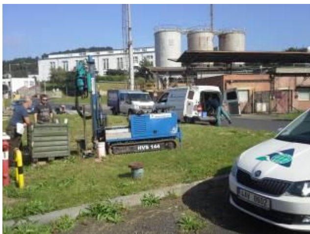
Figure 34: Soil sampling after injection (Source: AQUATEST a.s., Czech Republic)
