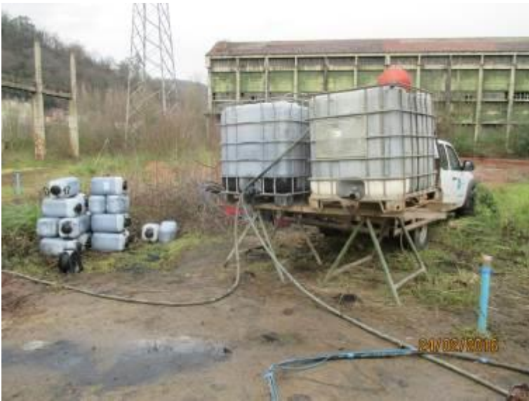
Figure 21: Empty containers and mixing tanks during nZVI injection application (Source: Fundacion Tecnalia Research & Innovation, Spain. Acknowledgements: Geoplano Consultores, S.A., Portugal & NANOIRON, s.r.o., Czech Republic)
