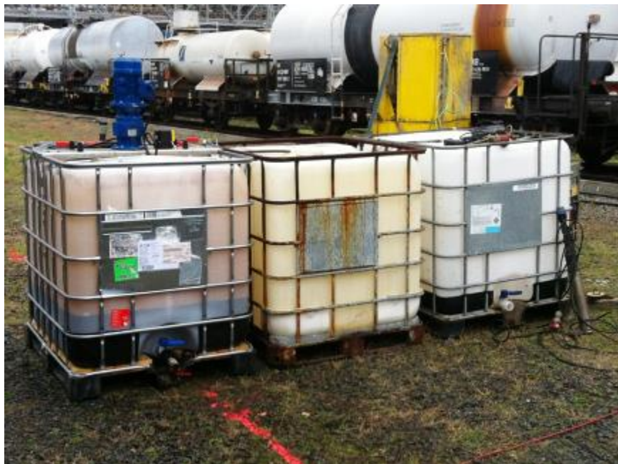
Figure 55: Deployment of Nano-Goethite nanoparticles for the injection at the SPOLCHEM site in Usti nad Labem (CZ) in November 2014 (left container: concentrated stock solution, right containers: containers for diluting the stock solution with water on-site). Injection was performed by AQUATEST on 18/11/14 (Source: University Duisburg-Essen, Germany)
