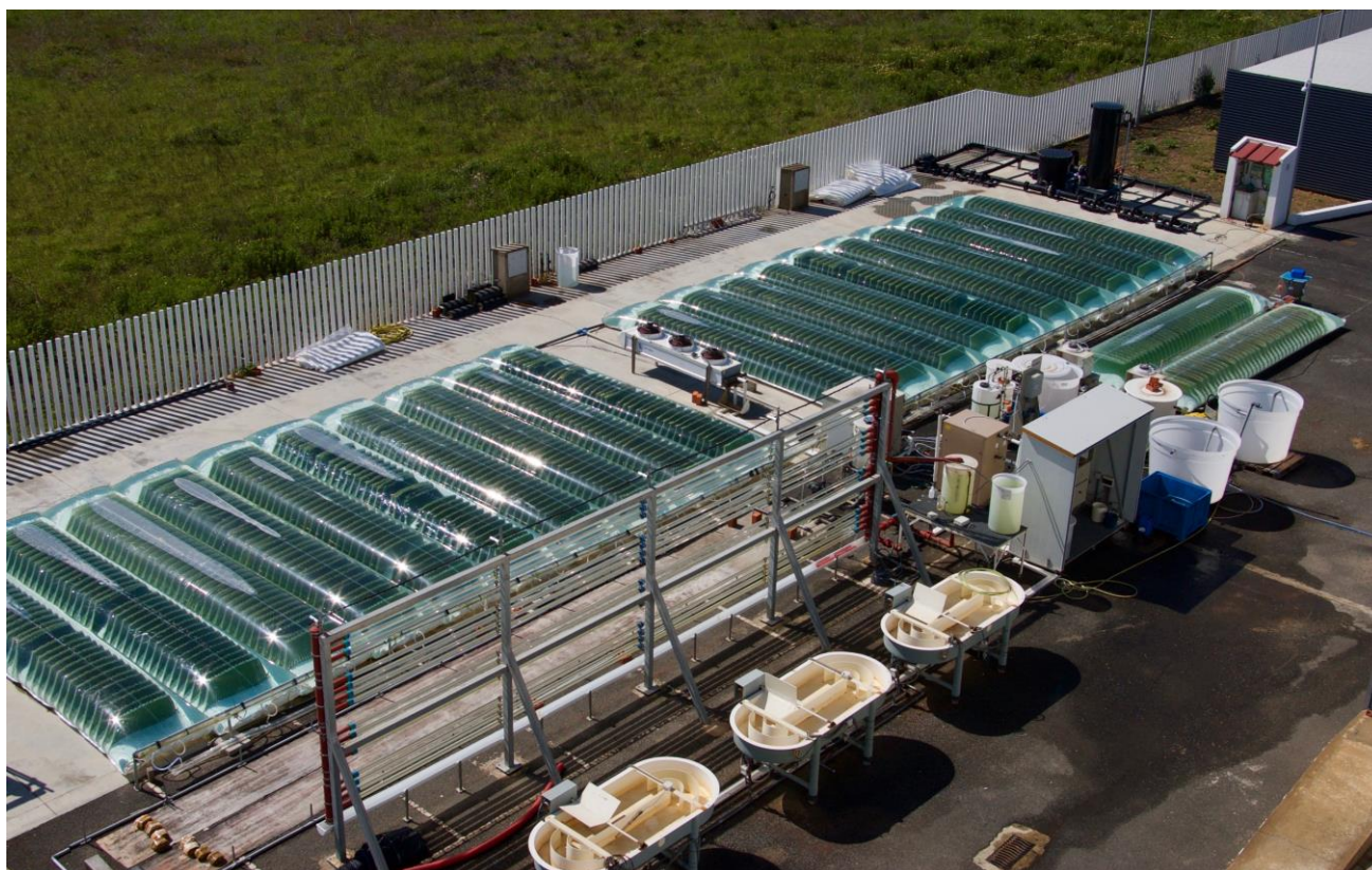
Figure 10. ProviAPT demonstration plant in Huelva, Spain at partner NIS
