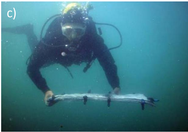
Figure 22. Use of carbon fibre impregnated with treated with cured epoxy-time enclosed in a plastic vacuum bag.
