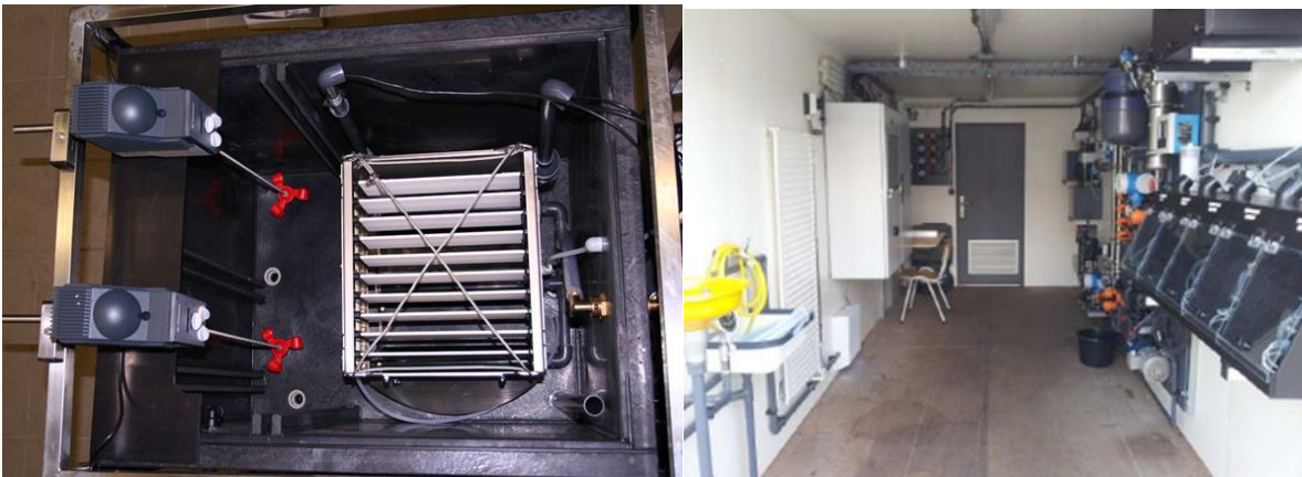
Top view of the plate and frame system of the HCMF demosites in Basel (left) and Almelo (right).
