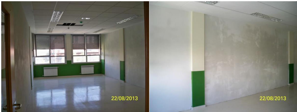
Figure 19: Installed plaster system in the test classroom.
