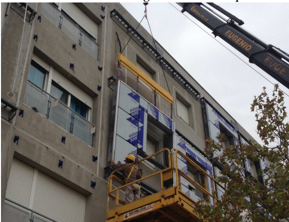
Figure 41. Fastening the Multifunctional Panels to the Structural Trays
