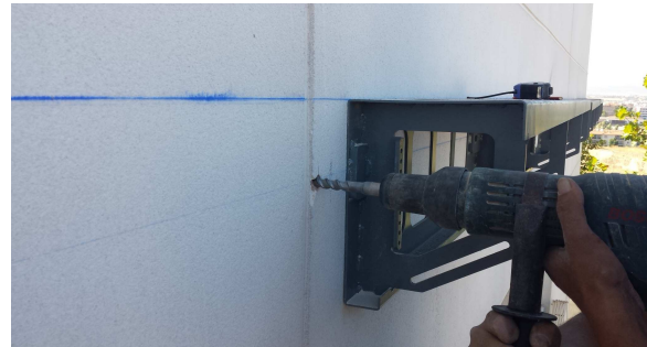
Figure 39. Installation of ETICS layer and fixing of Structural Trays
