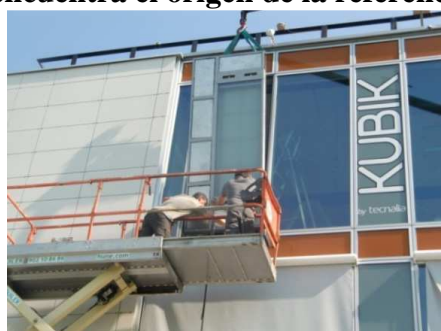
Figure15. Installation of the first prototype of the APSC&VU in KUBIK building
