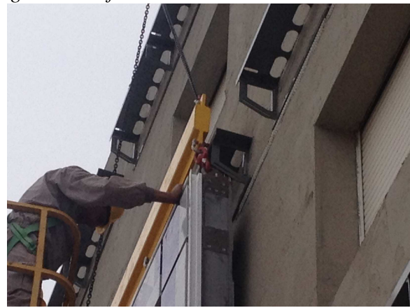
Figure 41. Fastening the Multifunctional Panels to the Structural Trays
