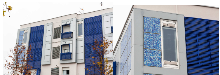
Figure 21. Detail view of one of the units
