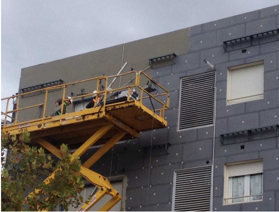
Figure 39. Installation of ETICS layer and fixing of Structural Trays
