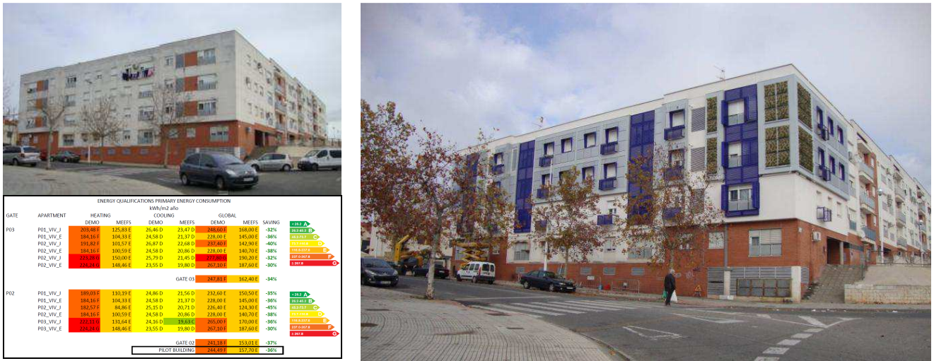
Figure 44. Pilot Building before and after the retrofitting with MeeFS System, on the left corner the final certification performed in comparison to the
