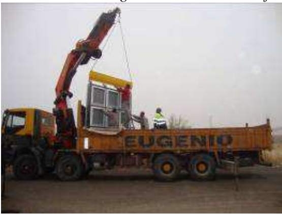
Figure 40. Transport and Lifting the Multifunctional Panels
