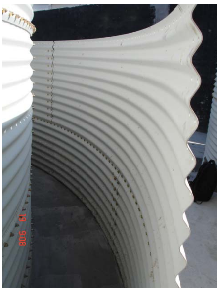
Photos 6 and 7. Detail of the corrugated galvanized sheet bolted steel and the double tank system
