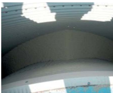
Photos 8 and 9. Detail of the insulation of the space between both metallic tanks and the bottom part.
