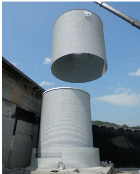
Photos 6 and 7. Detail of the corrugated galvanized sheet bolted steel and the double tank system
