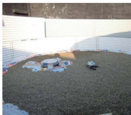
Photos 8 and 9. Detail of the insulation of the space between both metallic tanks and the bottom part.
