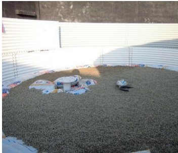
Photo 7. Bulk insulation of the tank bottom
