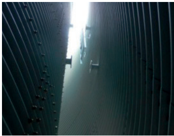
Photo 8. The chamber between two metallic layers.
