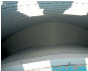
Photo 9. Insulation of the bottom of the STES
