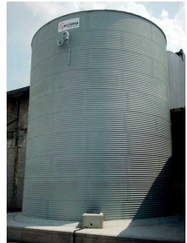
Photo 5. View of the STES in the Spanish Pilot Plant.
