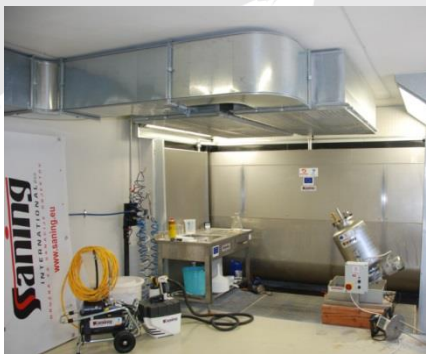
Fig. 6. Specially equipped chamber with multifunctional reactor for the consolidant pilot production
