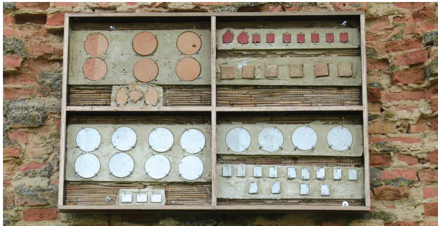
Fig. 12. Experimental panel for the assessment of the application techniques in the real environmental conditions, Bač Fortress
