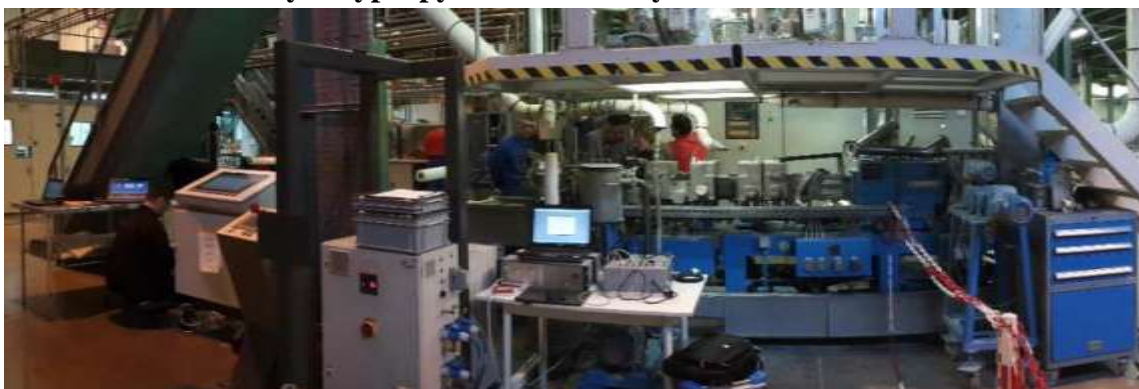
Figure 3.5.3.1 Extrusion line at Addiplast SAS.
