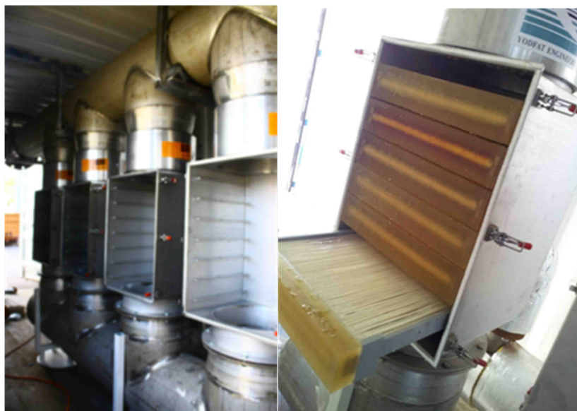
Figure 11 Empty trains including headers and one train filled with six modules
