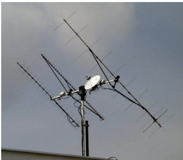
Part of antenna farm
