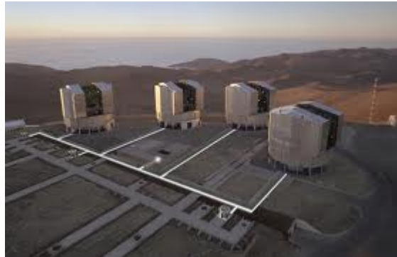
This image of the VLT at Paranal shows the tunnels which can be used when the four 8m telescopes are operated as an Interferometer (Photo ESO)
