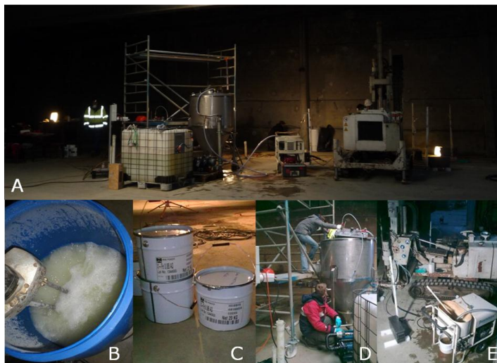
Figure 22. Iron injection set up. (A) injection area, (B) guar gum preparation, (C) mZVI, (D) mixing of guar gum and mZVI, (E) Geoprobe injection.
