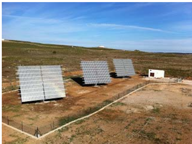
Fig. 3. Left: The CPV power station at IFRANE (AUI site) connectd to the utility grid of the partner ONE. Right: The cabin and house where the 6 inverters are installed. The site infrastructure has been provided by the associated partner AUI.
