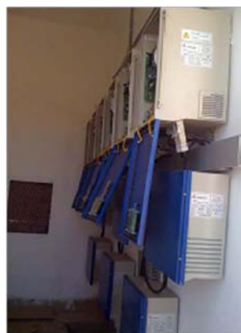
Fig. 3. Left: The CPV power station at IFRANE (AUI site) connectd to the utility grid of the partner ONE. Right: The cabin and house where the 6 inverters are installed. The site infrastructure has been provided by the associated partner AUI.
