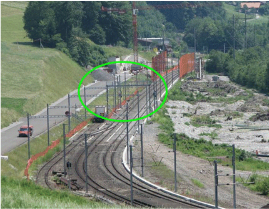
Fig. 1.3.4 Location of the Inspection Gate in Heustrich
