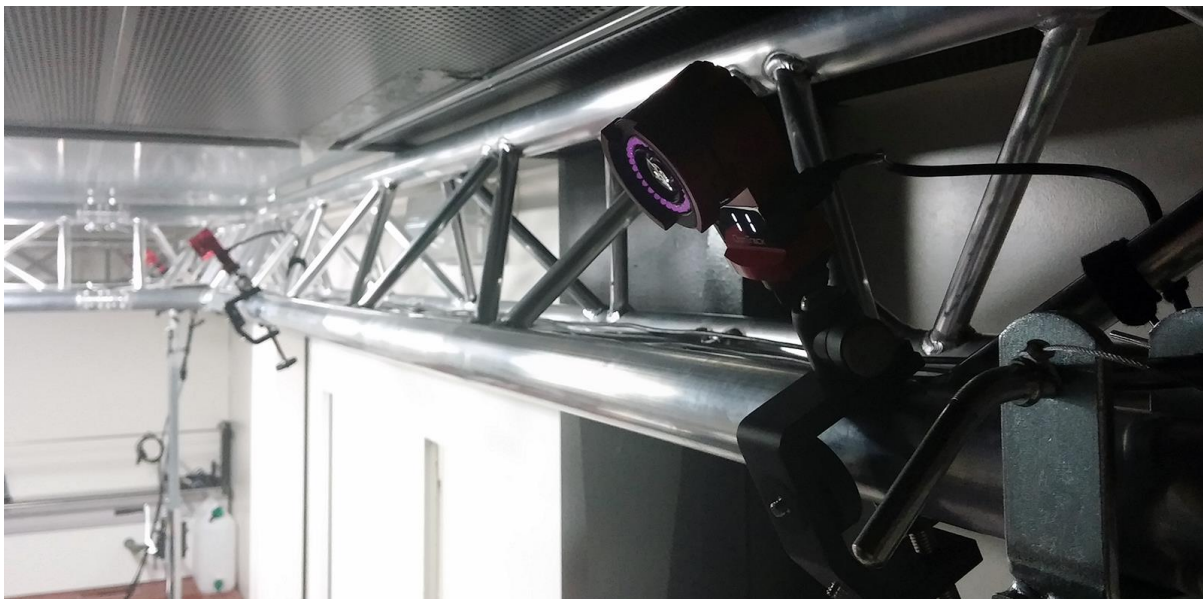
Figure 5.1: Optitrack Flex13 cameras mounted in the capture lab
