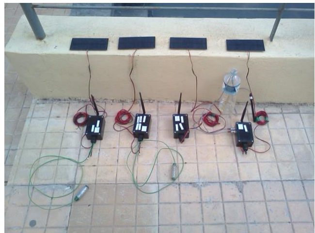
Figure 3-6: Sensors with solar panels
