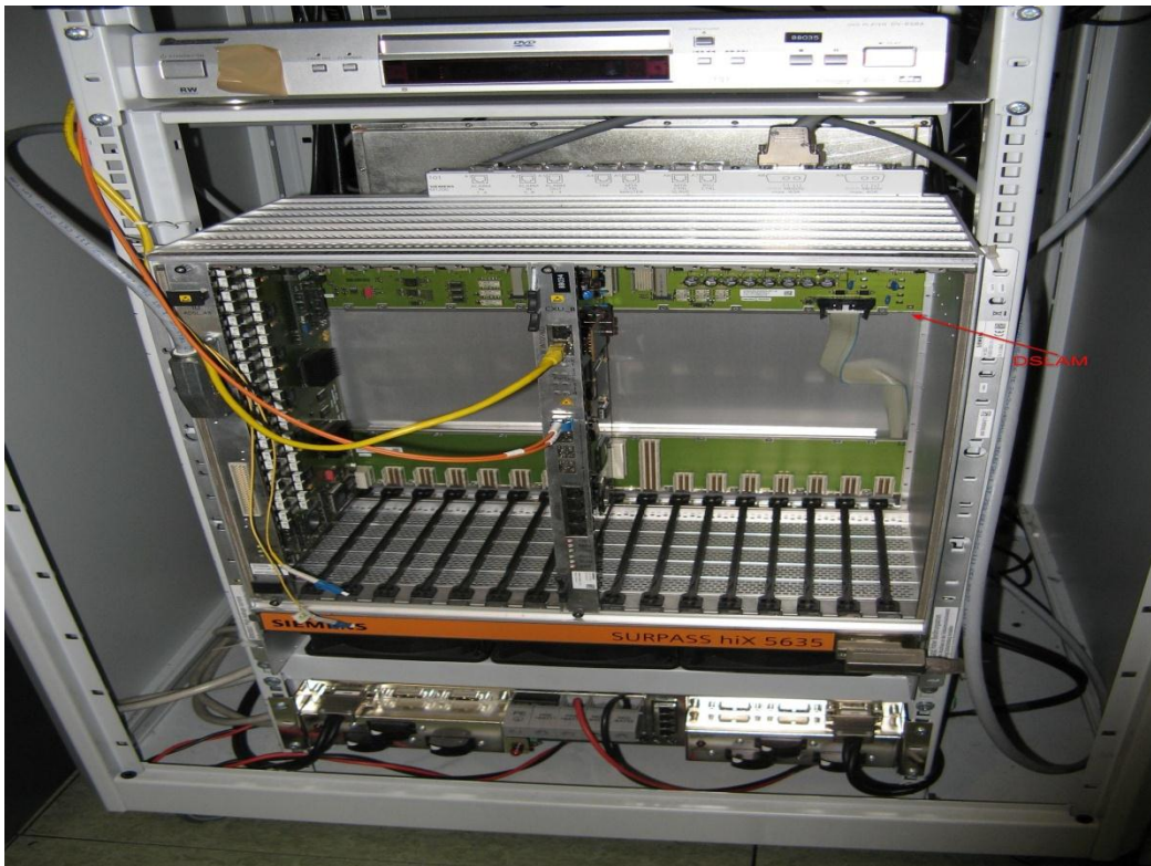
Figure 12: DSLAM (details)
