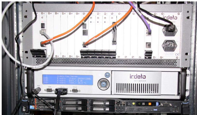
Figure 14: Encryption components: IRD IPTV Scrambler, IRD KeyServer, and IRD KMS
