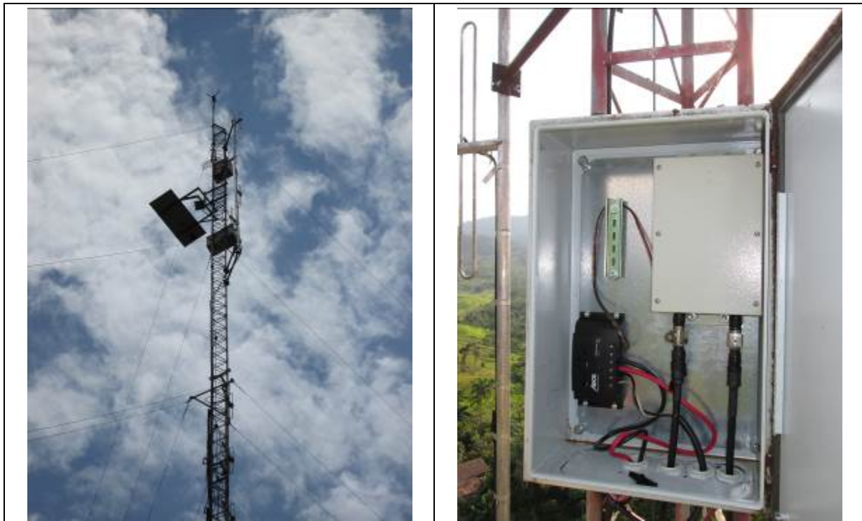
Figure 57: Maintenance of the equipment used in the repeater located in Balsapuerto.
