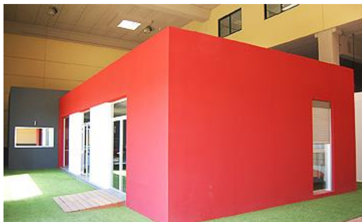
Figure 30 Exterior picture of the CIAMI Living Lab
